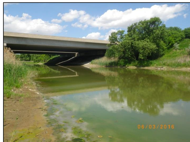
H1: Facing north (upstream) from the runningway (Spring 2016).
