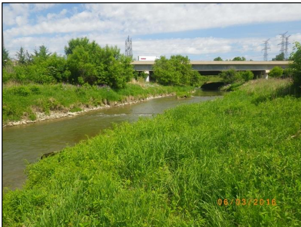
H7: Facing north (upstream) from the runningway (Spring 2016).
