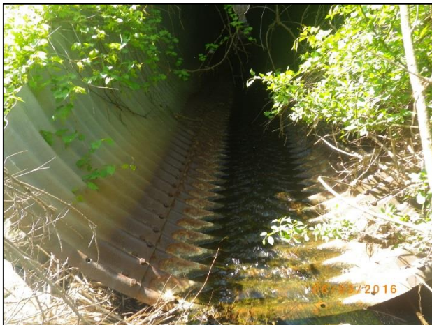
H8: Facing south (downstream) from the CNR (Spring 2016).
