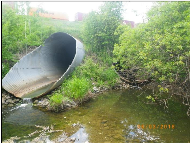
M5/6: Facing west (upstream) from east of the CNR (Spring 2016).
