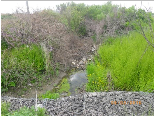
M3: Facing north (upstream) from the hydro access road (Spring 2016).
