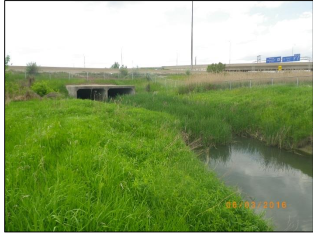
M4: Facing north (upstream) from the runningway (Spring 2016).
