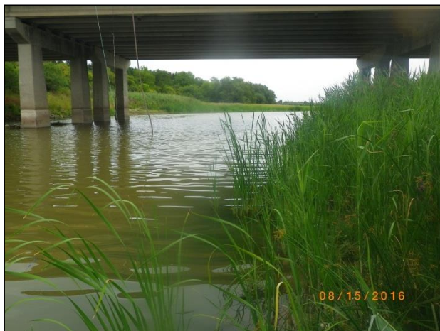
H1: Facing south (downstream) from the runningway (Summer 2016).
