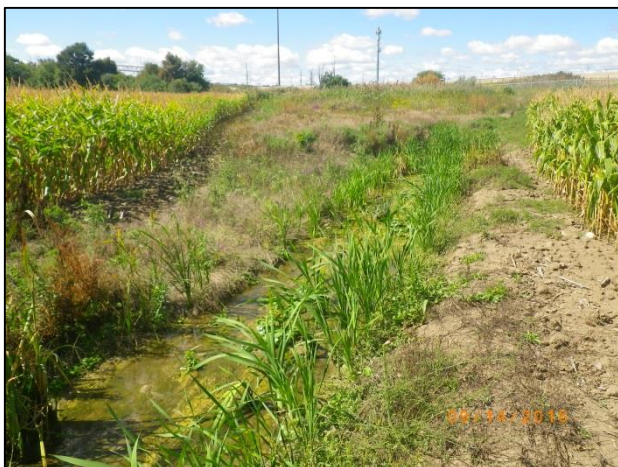
E3: Facing north (upstream) from the runningway (Summer 2016).
