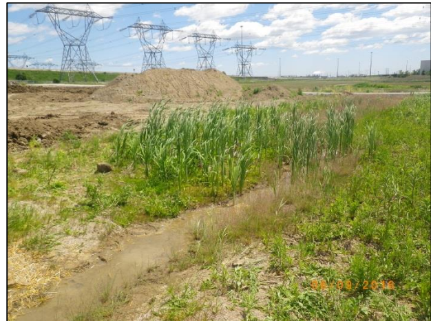
E4: Facing south (downstream) from the runningway (Spring 2016).
